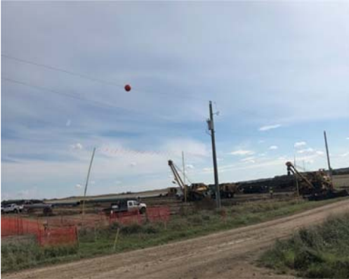
SF 28 photo facing south east, two side booms moving the welder that goes inside the pipe across the road.
