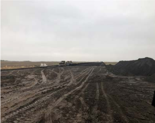
SF 14, photo facing west, speed dozer being pulled by dozer pushing topsoil, one grader grading the ROW.
