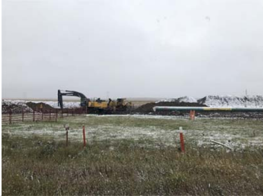
SF 24, photo facing east, coating crew on sight coating the weld on the pipe.
