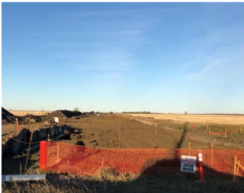
SF 4, photo facing west, one grader grading and one dozer pushing soil.
