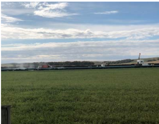
SF 27, photo facing south. Coating crew coating the pipe.
