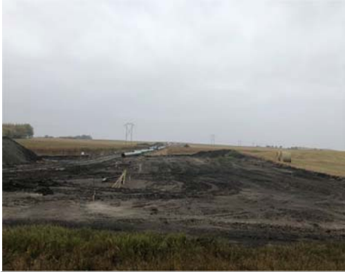
SF 30, photo facing west, pipe gang working on the pipe off in the distance, ROW was very wet and muddy.
