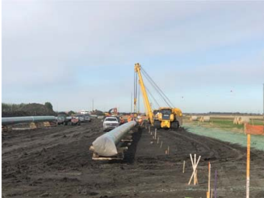
SF 24, photo facing west, crews jeeping the pipe.
