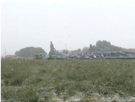
SF 27, photo facing south, crews spraying mulch off the back of the truck onto the north side of the ROW.
