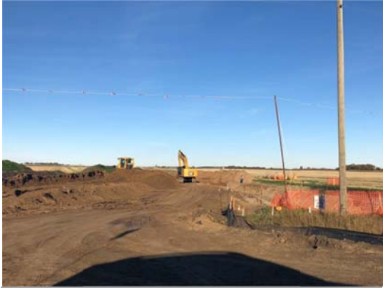
SF 7, photo facing west, excavator and dozer backfilling pipe.
