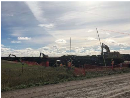
SF 5, photo facing east, crews backfilling pipe.
