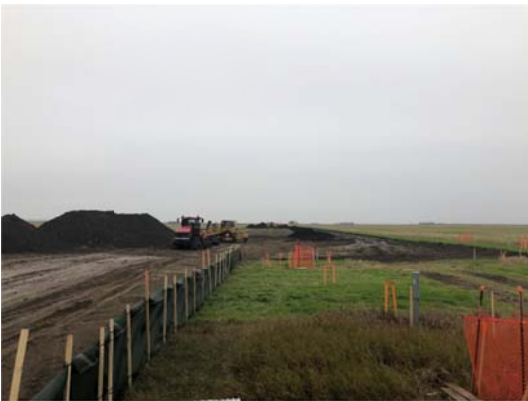
SF 14, photo facing east, 11 dozers total all striping top soil pushing it to the side of the ROW.
