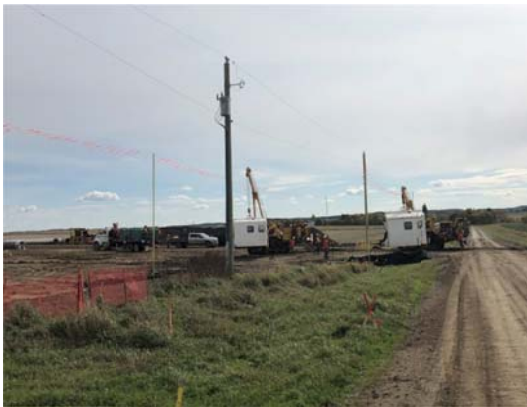
SF 28, photo facing south, pipe gang crew moving welding shacks across the road, flaggers were used.
