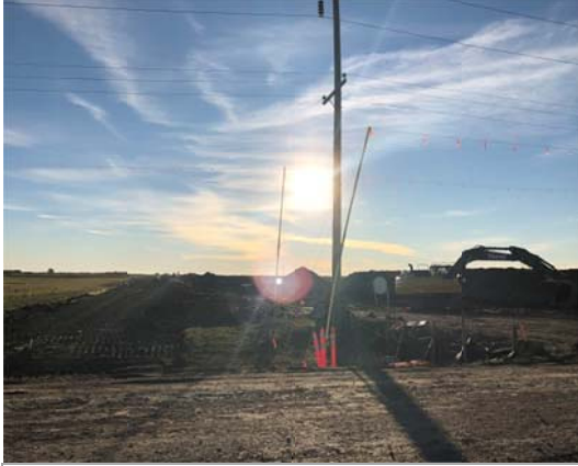
SF 4, photo facing east, crews packing dirt on the ROW.
