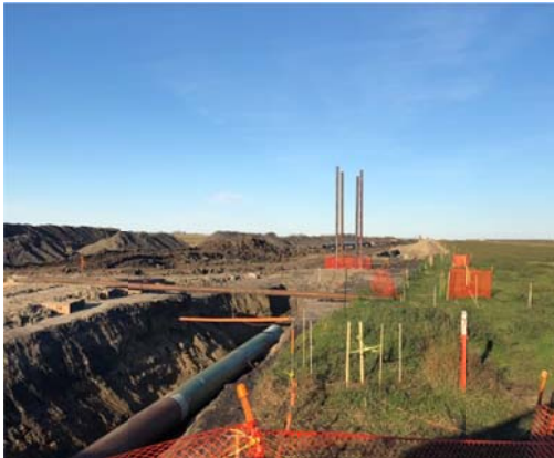
SF 5, photo facing west, three excavators back filling pipe, (excavators are a little hard to see)
