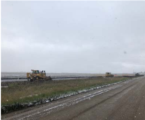
SF 17, photo facing north east, 2 dozers stripping soil.
