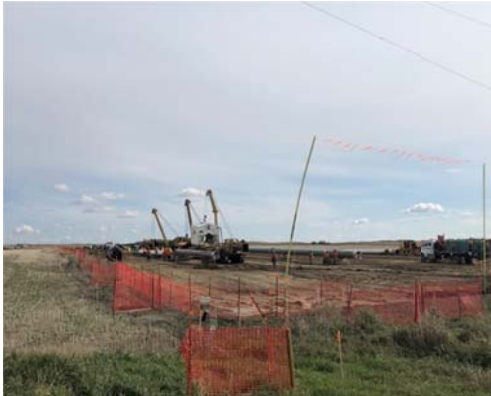
SF 28, photo facing south east, pipe gang crew welding pipe together.
