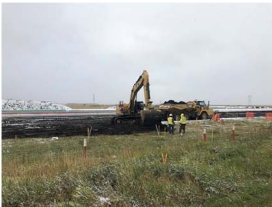
SF 22, photo facing south, one excavator digging soil loading it into the back of the rock truck.
