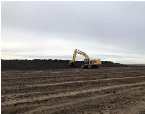
SF 17, photo facing south west, excavator smoothing down transition pile with the back of his bucket.
